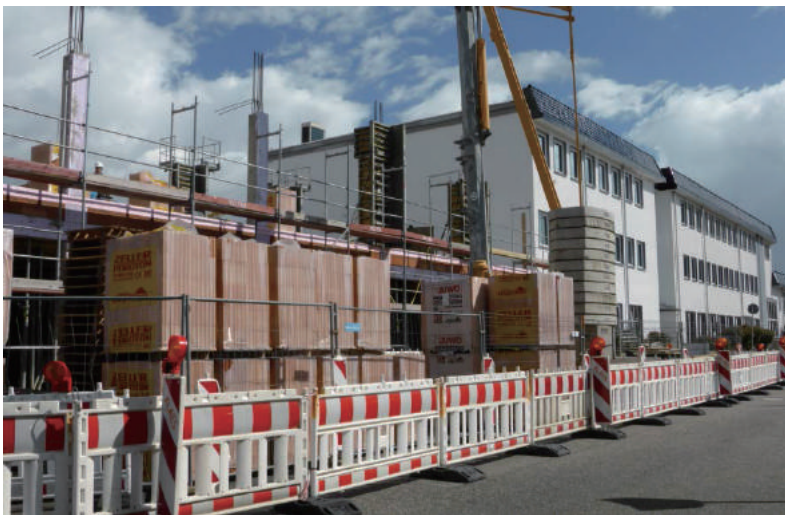
Construction site at the Giessen location
